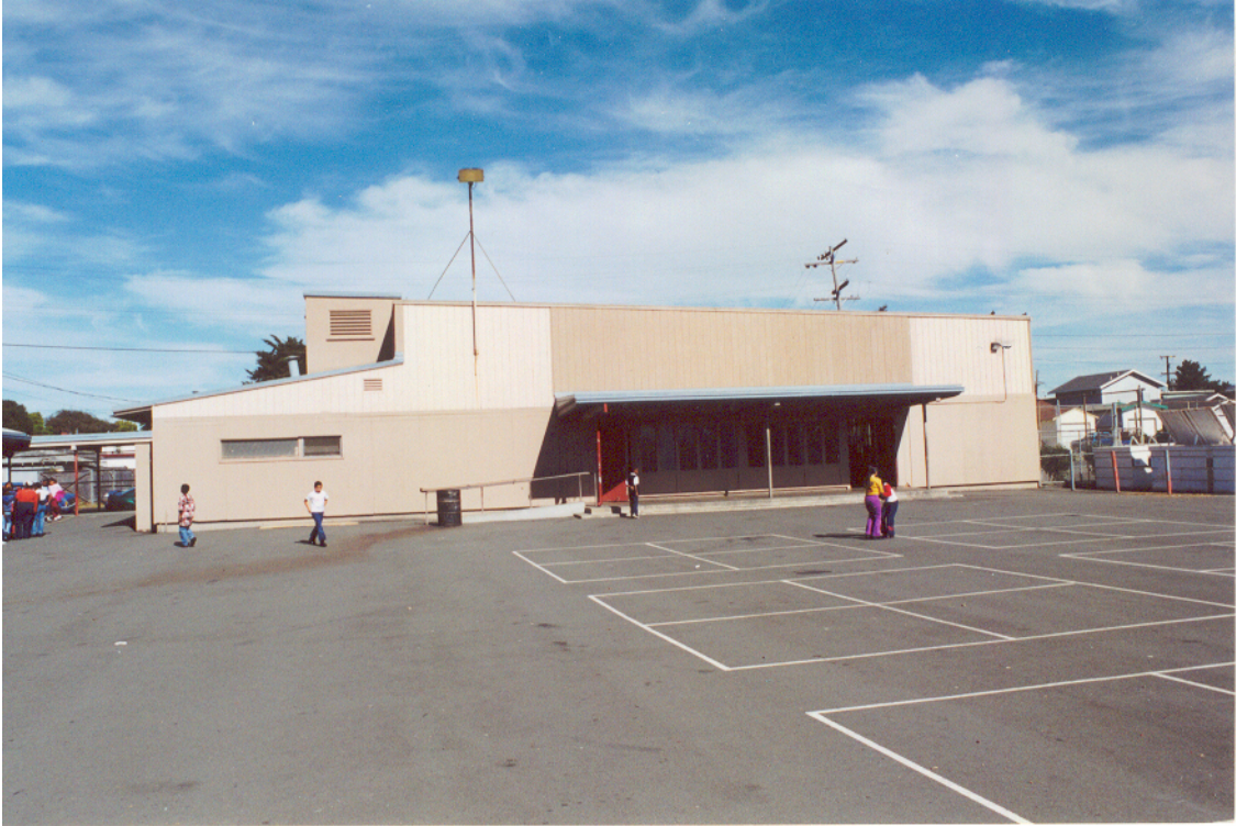
Figure 22: Northwest Face of Multi-Purpose Building
