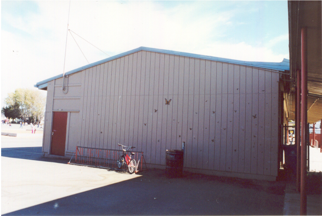
Figure 5: Northeast Face of Kindergarten Building
