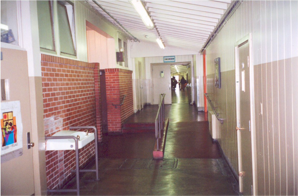
Figure 15: Corridor between Classroom Buildings at Restrooms
