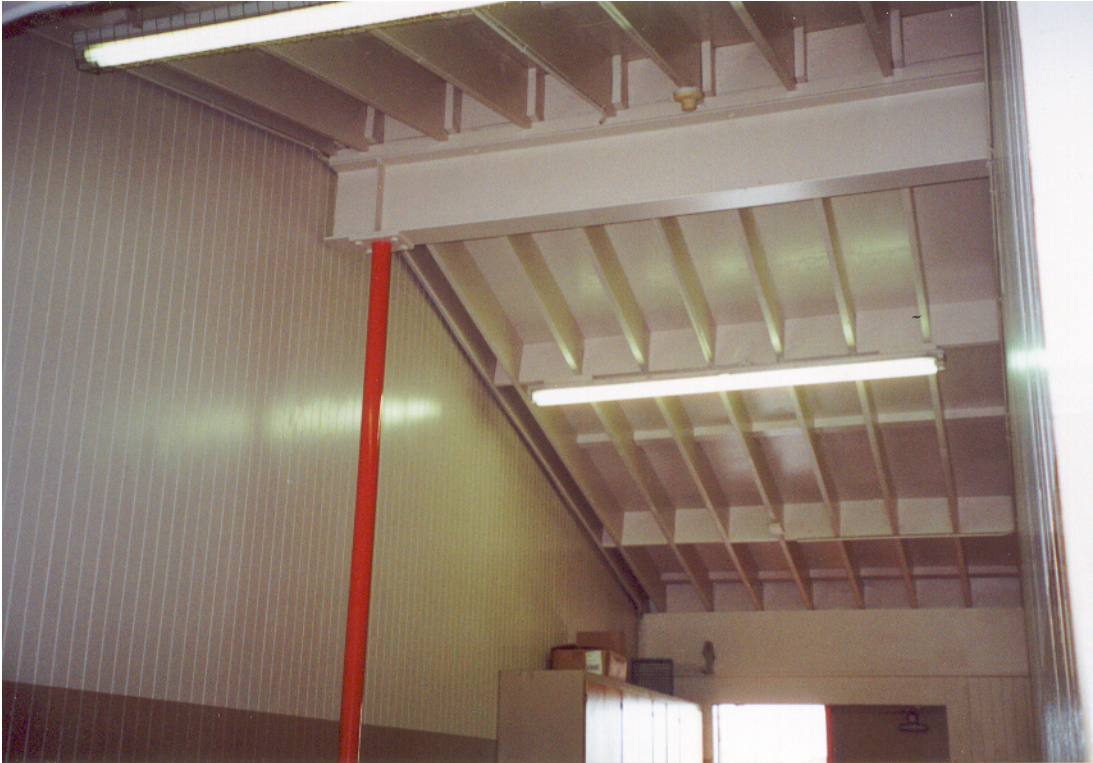
Figure 16: Corridor between 1960 and 1962 Classroom Buildings
