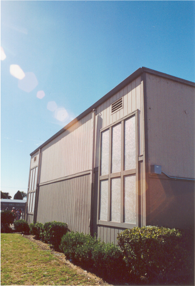
Figure 23: Southwest Face of Multi-Purpose Building
