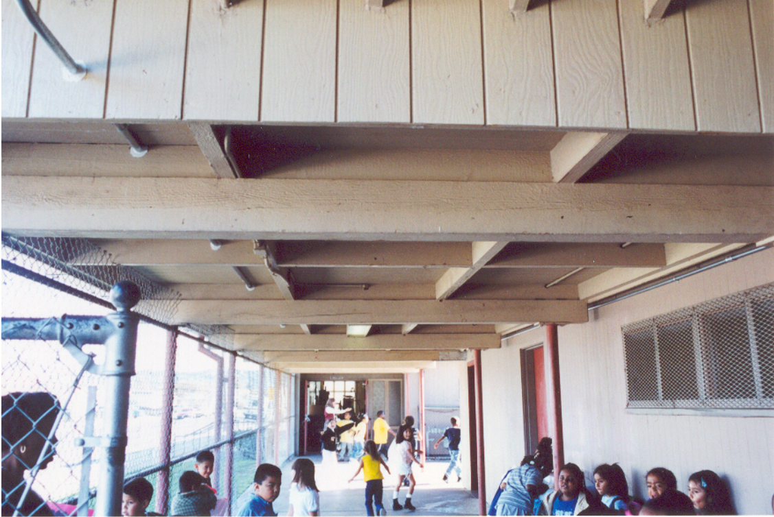
Figure 18: Covered Walkway at Southeast End of Classroom Buildings
