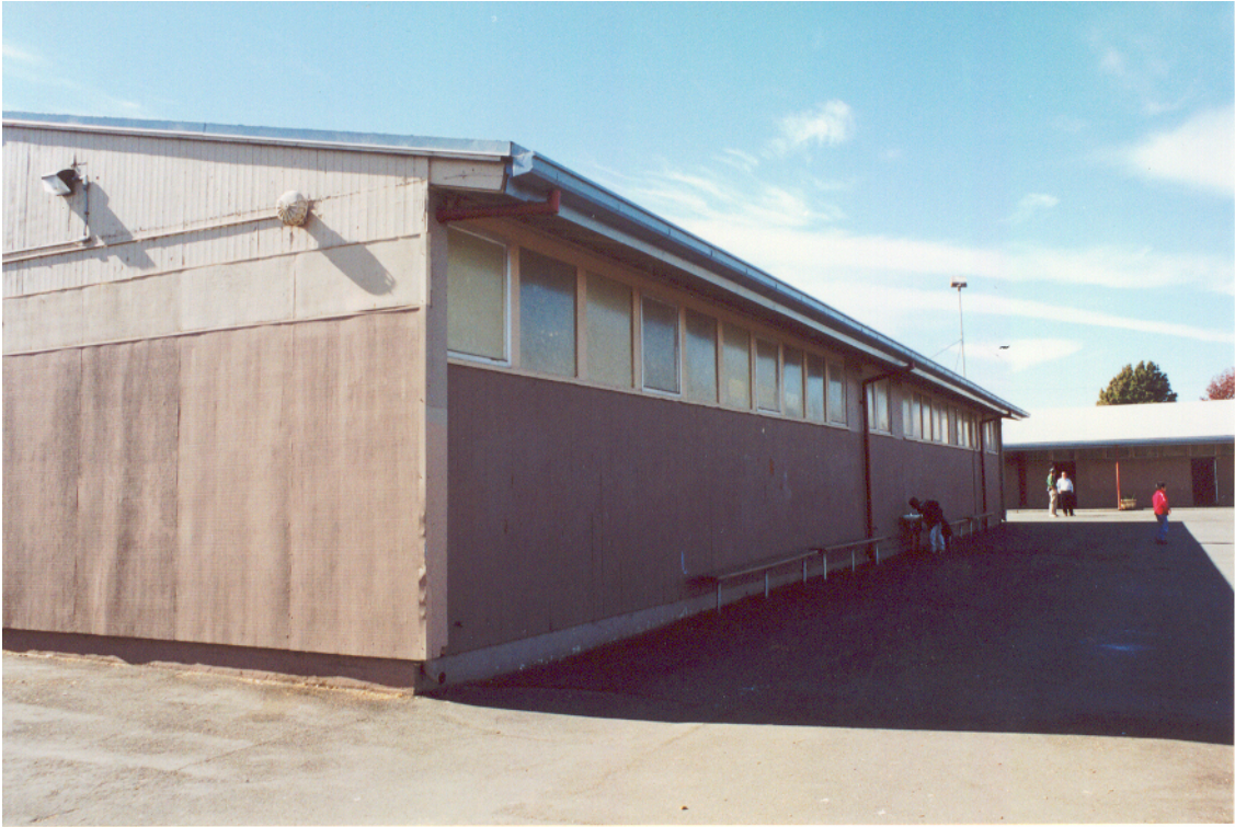
Figure 9: Southeast Face of Kindergarten Building
