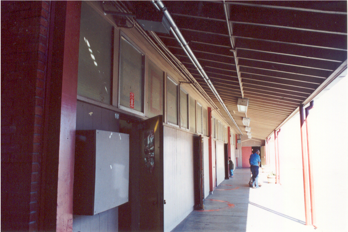
Figure 12: Southwest Face of 1952 Classroom Building
