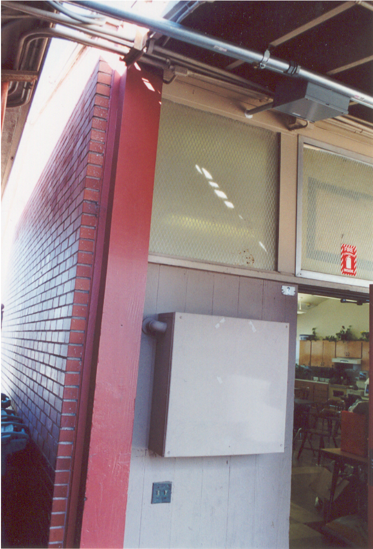
Figure 11: Seismic Joint between Office Building and 1952 Classroom Building
