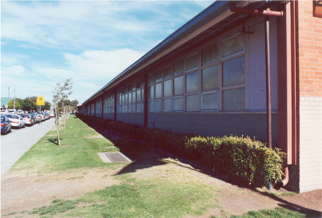
Figure 10: Northeast Face of 1952 Classroom Building
