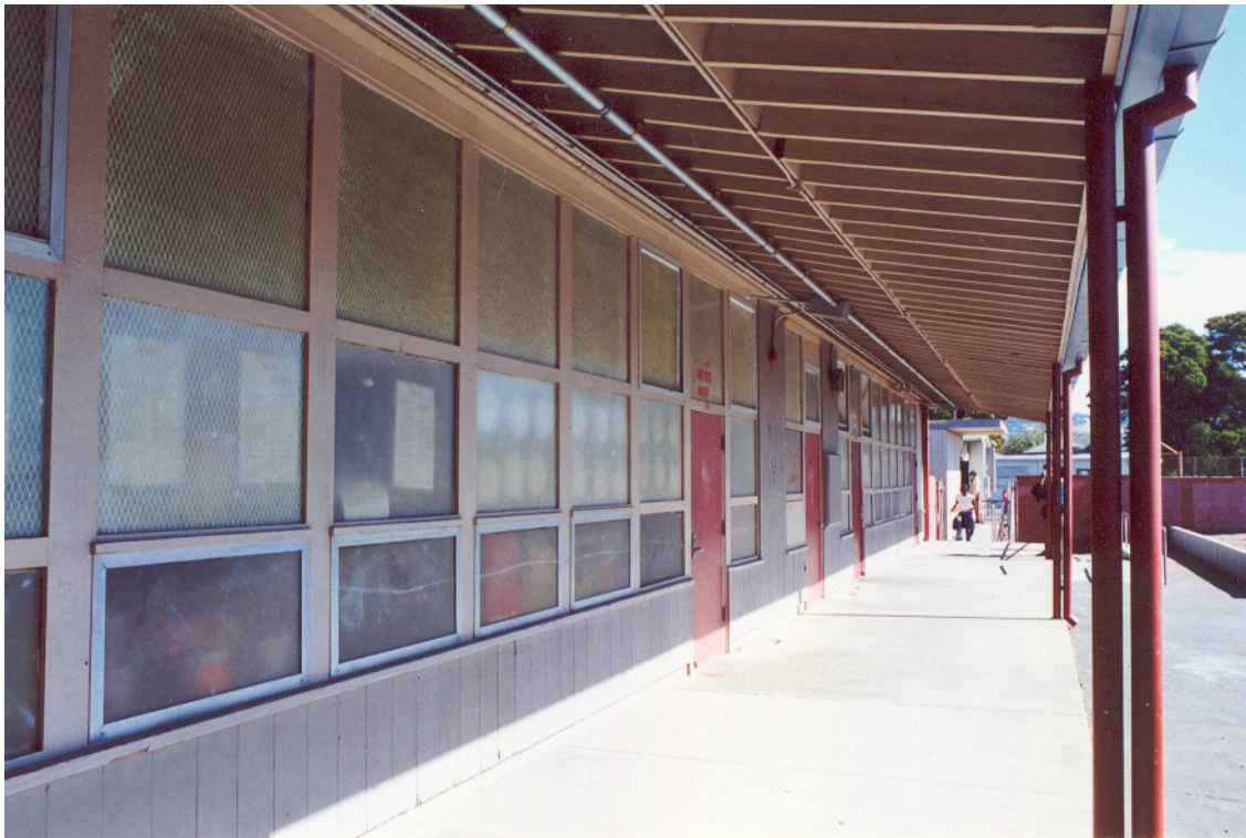
Figure 6: Northwest Face of Kindergarten Building
