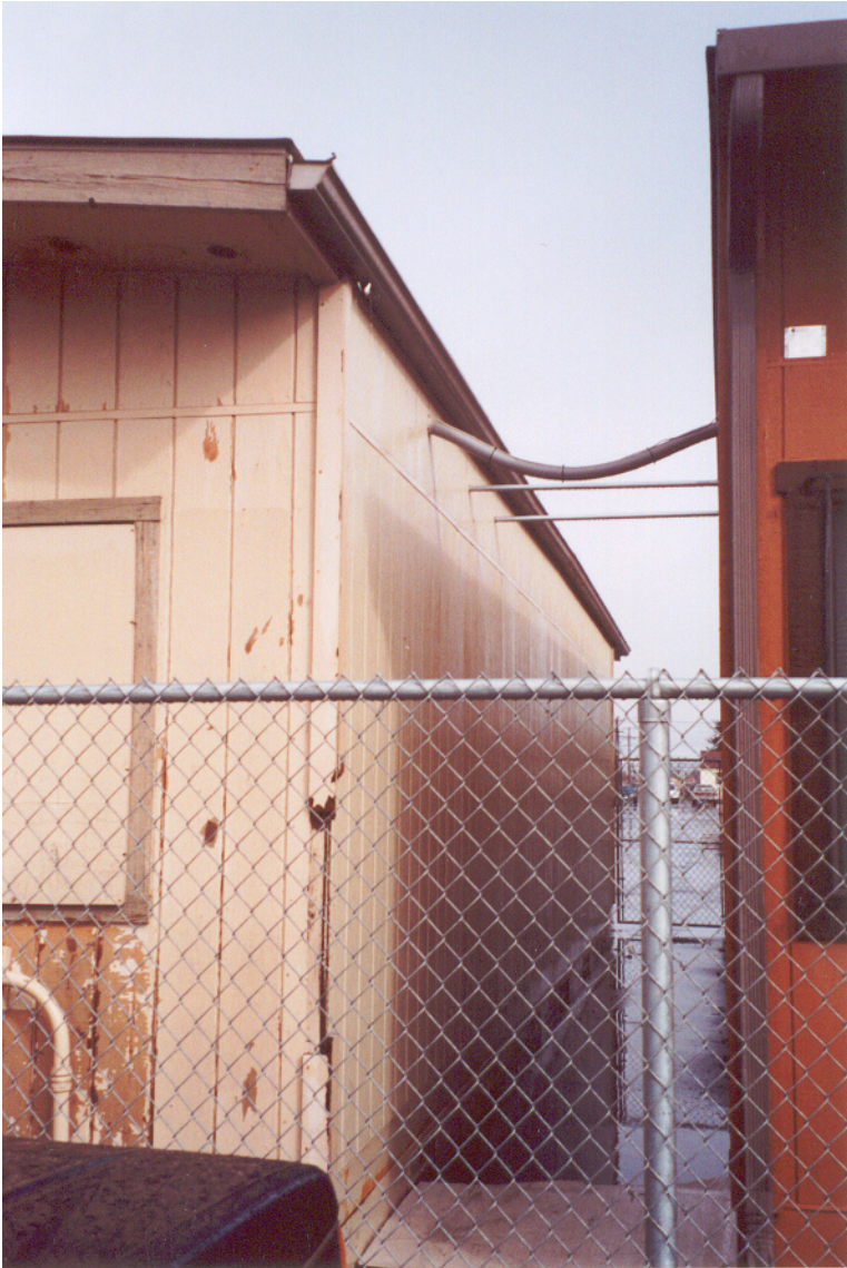
Figure 24: Conduit between Portable Units
