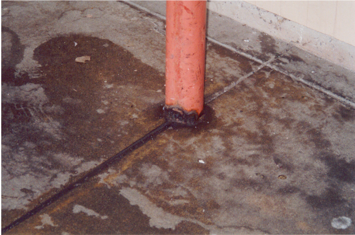
Figure 20: Rust at Covered Walkway Column
