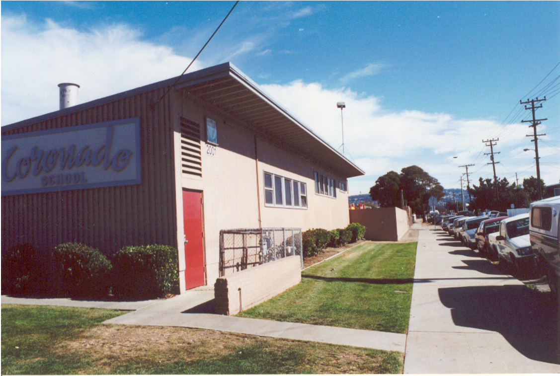
Figure 3: North Corner of Office Building
