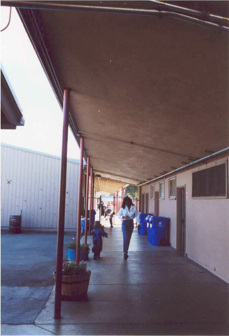
Figure 4: Southeast Face of Office Building
