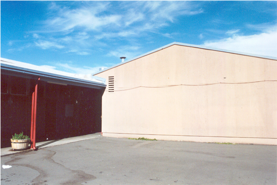
Figure 13: Northwest Face of 1962 Classroom Building at 1952 Classroom Building
